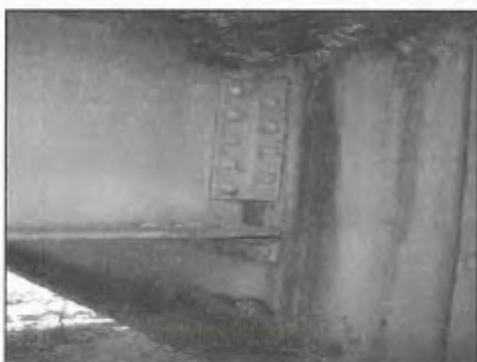
Figure B-17—Corrosion at Floor Beam Ends
