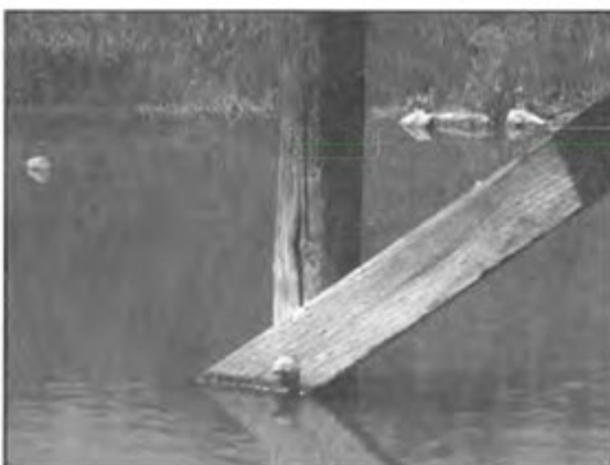
Figure B-4-7-in. Deep Check in Right Exterior Pile of Bent 2
