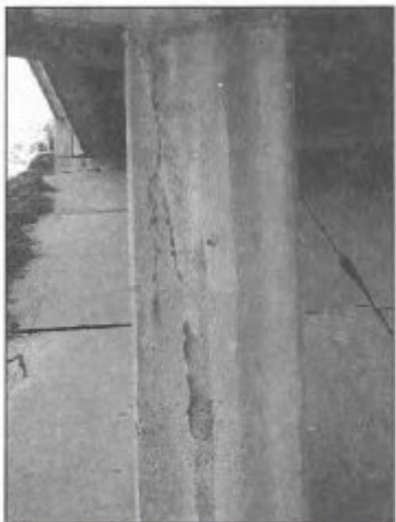
Figure B-12— \frac{3}{16} -in. Width Vertical Crack in Left Column of Pier 4
