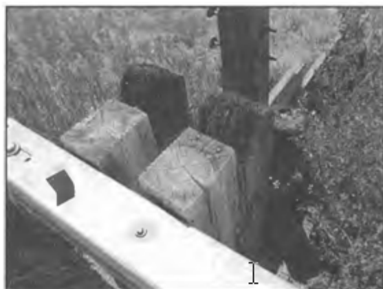
Figure B-5-Decay in Timber Rail Posts
