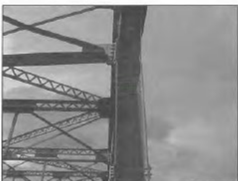
Figure B-15—Sway Bracing Impact Damage in Span 1
